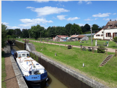
double sluice of Mont- et- Marré
